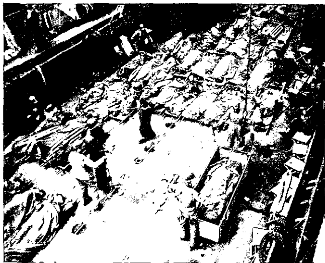
Figure 217. Loading large landing craft (LST) by use of loading box (France).
